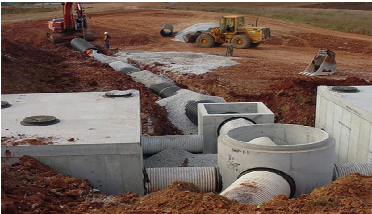
Figure 8. Another view of installation of storm water treatment bunkers and supply pipeline at Kentucky Transpark, Bowling Green, KY (Photo courtesy of Contech Engineered Solutions, http://www.conteches.com/DesktopModules/Bring2mind/DMX/Download.aspx?EntryId=750 )
