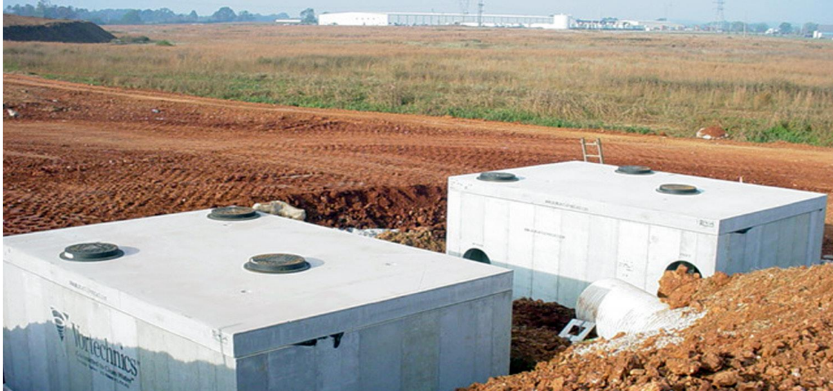
Figure 7. Photograph of installation of storm water treatment bunkers at Kentucky Transpark, Bowling Green, KY (Photo courtesy of Contech Engineered Solutions, http://www.conteches.com/DesktopModules/Bring2mind/DMX/Download.aspx?EntryId=750 )
