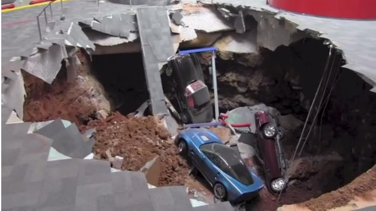
Figure 17. Photograph of sinkhole collapse at National Corvette Museum (Photo Courtesy of National Corvette Museum).
